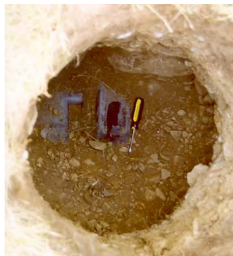
Fig. 3.5 Hand excavation from ground
